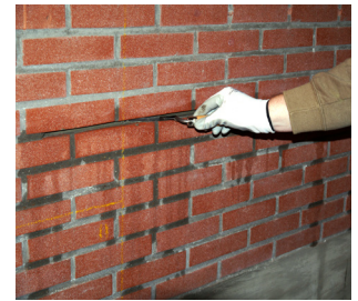
Push the bar into the grout and then inject another bead of grout
