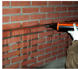
Injecting the bead of grout
