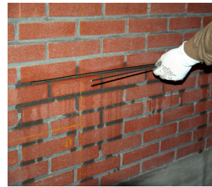
Laying in the bar
