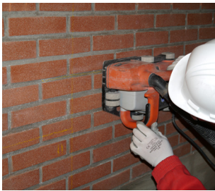
Chasing the wall
