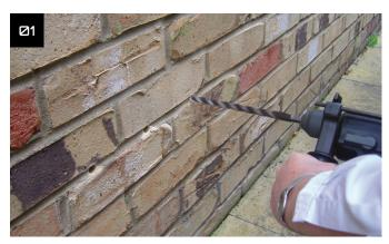
12mm diameter holes drilled horizontally into the mortar joint at 120mm centres and to a depth of 10 - 20mm from the opposite face.
