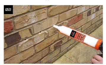
Fill drilled holes with SAMSON DAMP-TECH® Injection Cream using a standard mastic gun, and make good with matching mortar.
